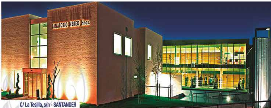
C/ La Tesilla, s/n - SANTANDER GPS: N 43° 27' 53.56" W -3° 50' 4.80"
